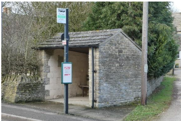
Bus stop on Main Road
